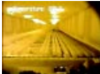
Steel reheat furnace
